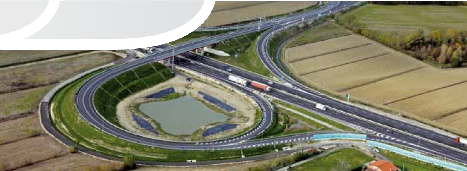
Impregilo - A4 Motorway project in Mestre, Venice
