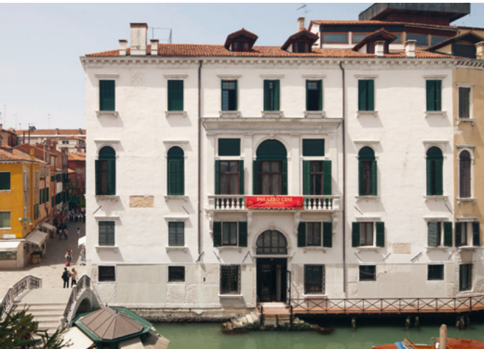
Above: Palazzo Cini, seen from Campo San Vio. ©Matteo De Fina
